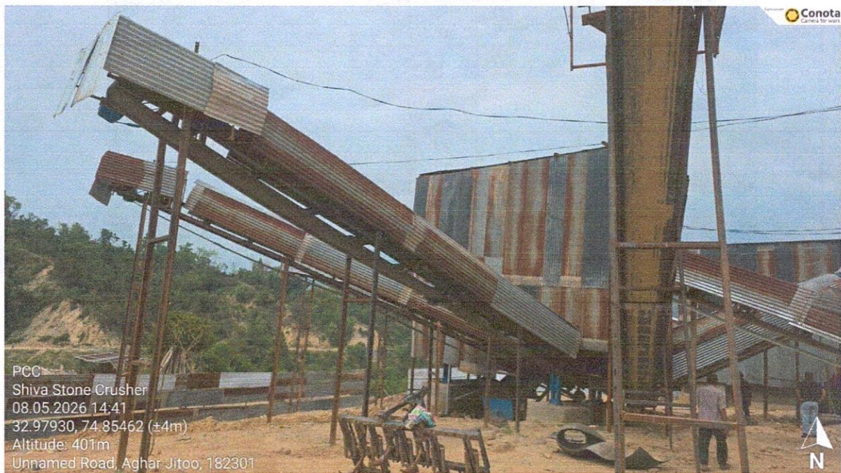
Pic-2: Conveyor Belts covered with GI Sheets
